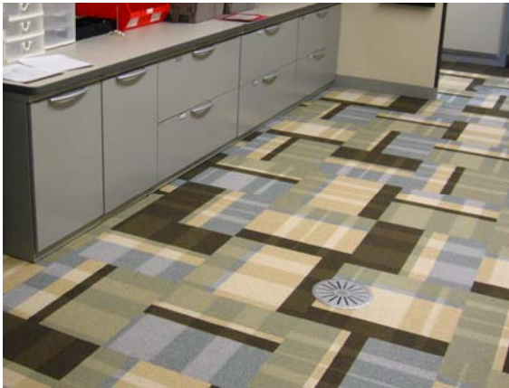
Figure 2: Under-floor air distribution in CDC
