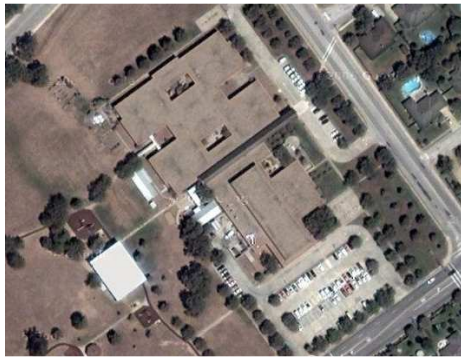
Figure 8: Satellite view of the case study school building
